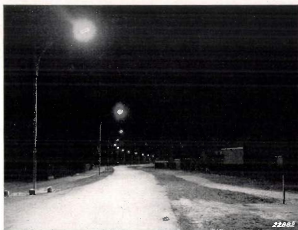
Fig. 3. Example showing the importance of illuminating the areas skirting country roads in addition to the road itself, so as to obtain a sufficiently extensive background. It may be seen how each of the traffic lanes produces its own particular brightness stimulus.
