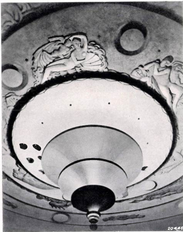
Fig. 8. The giant candelabrum of the Roxy Theatre in New York is not only an interesting lighting ornament, but also reveals shadow edges and decorative bas-relief which are only brought out by the grazing light rays.
