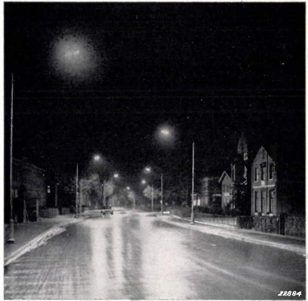
Fig. 13. Transverse light sources with large radiating surfaces produce wide luminous bands with a comparatively low brightness on a wet road surface.
