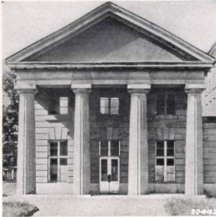
Fig. 1. (Left) A building in the Doric style as seen in sunlight. All forms and profiles stand out with their true values. It is distinctly seen how e.g. the flutings and the cornice have been designed entirely on the marked contrast between light and shadow.
